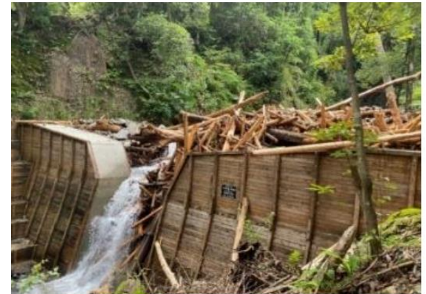
A driftwood-catching dam (Kuma-mura, Kumamoto Prefecture)
